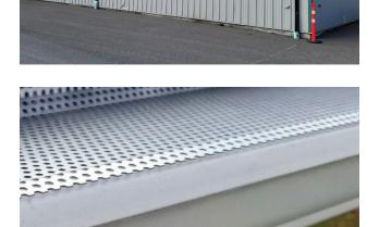
for metal roofs lacking snow guards. Without these guards, heavy snowfall can cause significant damage, potentially ripping off gutters. Our wrap-around hangers effectively mitigate snow load on metal roofs
